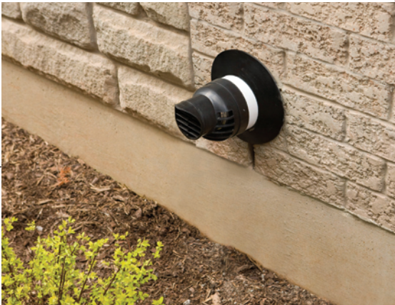
► The single concentric vent acts as both an air intake and exhaust, greatly simplifying installation.
