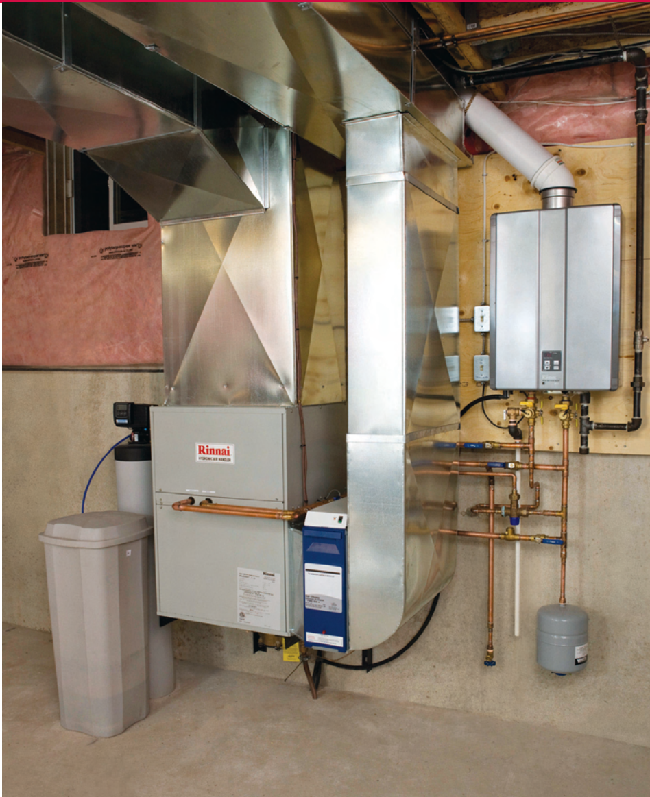
▲ Neat, compact installation moves the typical space-hogging furnace and water tank combo from the centre of the room over to an outside wall saving about 25 feet of floor space.
